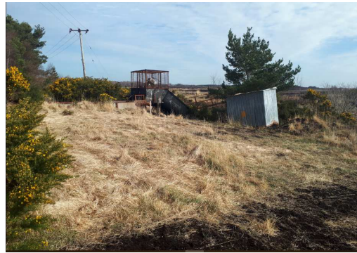
Photo 5.9.2 - Pump Site, Glashabaun North
