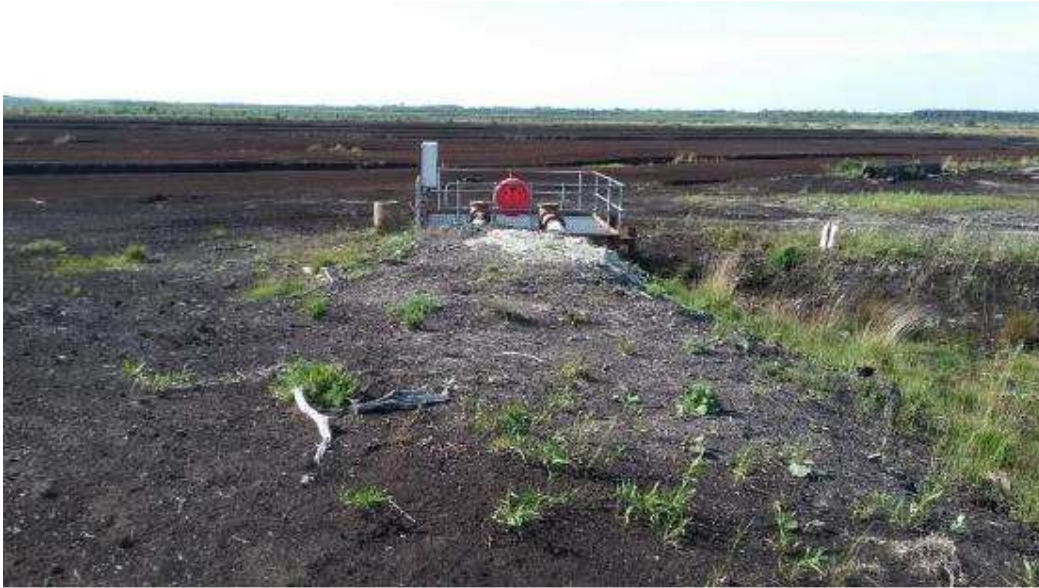
Photo 1.3.3 - Typical Submersible Pump Sump
