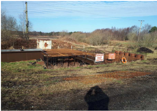
Photo 5.9.1 - Pump Site, Ticknevin
