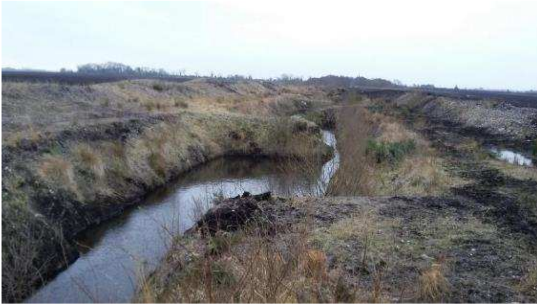
Photo 1.3.1 - Typical Example of Silt Pond
